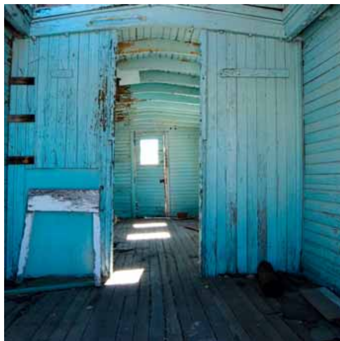
Boxcar © Josh Kellogg, 2008 First Place Windows/Doors Category CCCC Competition, October, 2008
